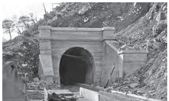
The Otira tunnel in 1910 during construction
